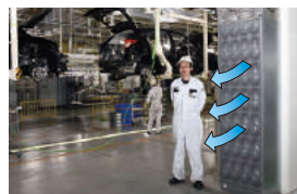
Air diffuser installed on the lower end of a pillar inside the factory
