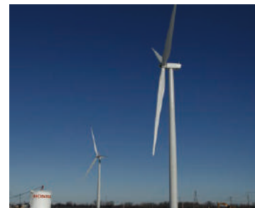
Two 1.7 MW wind turbines provide about 10% of the plant's electrical needs
