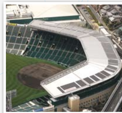
The Hanshin Koshien Stadium is equipped with thinfilm solar panels manufactured by Honda Soltec.
